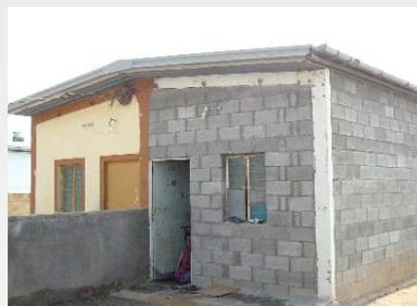
Picture 4. A reconstructed house with a steel frame and concrete blocks.
