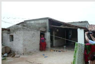
Picture 3. Expansion of a reconstructed house using conventional construction methods (left part)
