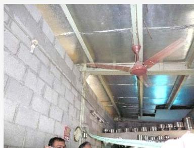
Picture 5. The top of the block wall is not attached to the structural members
