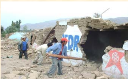
Demolition of damaged houses for reconstruction
