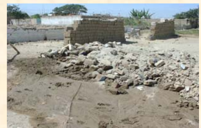
Recycle adobe rubbles for construction
