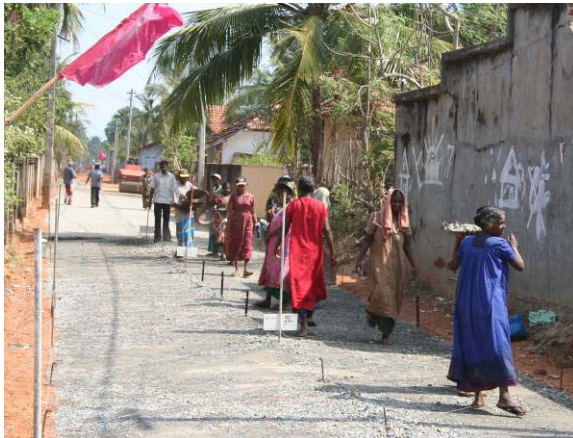
Photo 3: Placing base course using strings, pegs & line levels for layer thickness & camber control
