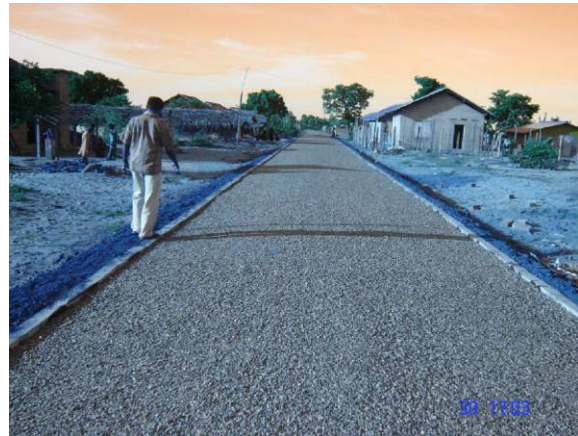
Photo 4: Completed road section
