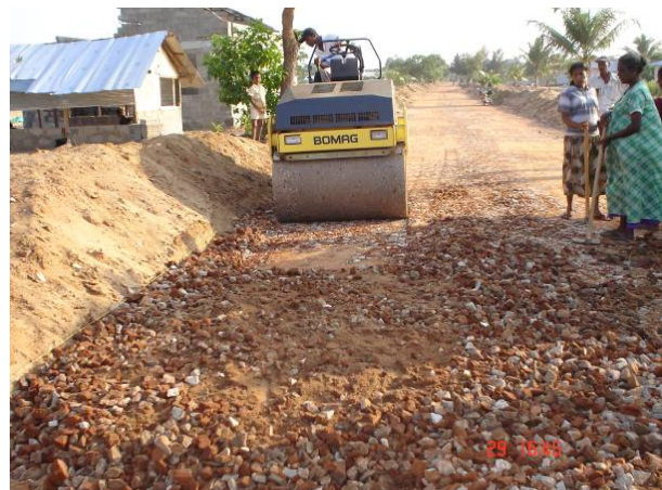
Photo 2: Compacting crushed and blended tsunami debris for sub-base layers.
