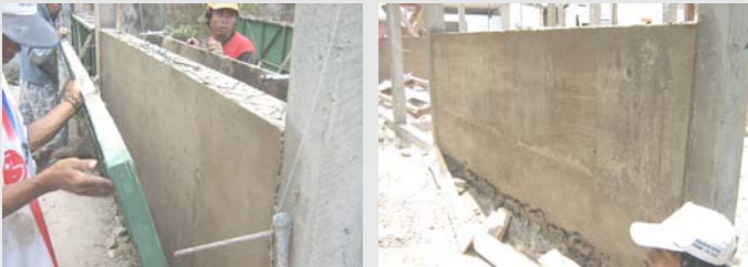
Figure 4. Frame works can be dismantled after one day.
