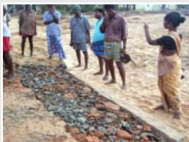
Changing roles is possible: supervising community infrastructure repairs.
